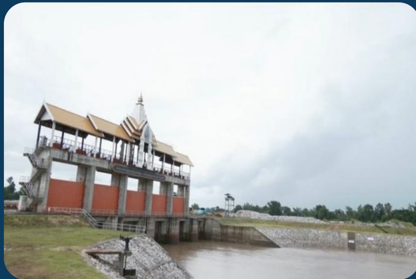
Lam Nam Pheung-Nam Kam Floodgate
